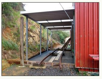
Chris and his crew continue with progress on this. During the last working bee they compacted some crusher dust into the floor area. They also bent some of the rails that will form the siding into the shed.
