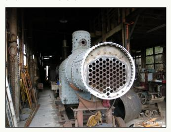
The welder was up from Wellington for a week working on the boiler. Some rivets were put in the dome and the new tube plate welded in.
