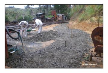
Chris Lucas and his crew are still progressing with this job. They are presently boxing up the shed floor area. They propose to lay the rails then mix and pour the concrete. A truck load of metal for the siding has arrived and is partly in place.
