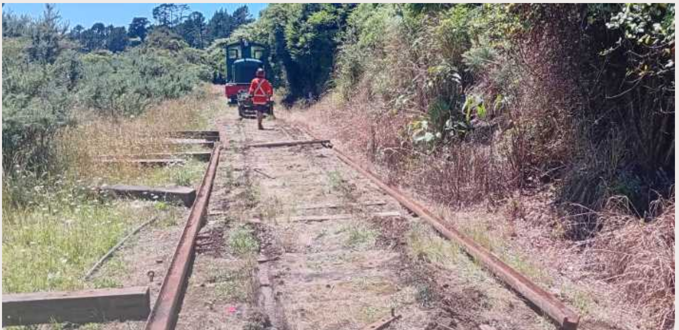
Above: Track reinstatement up the line near 1750m (Mike A)
