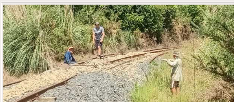
Above: Track work in January (Mike A)
