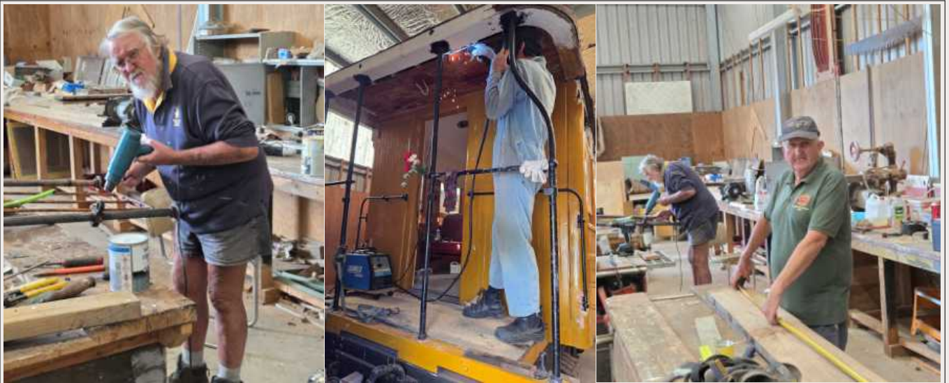
Above: Work progresses on the No.3 car – from left, Russ W, Trevor T, Bruce McL (Richard E)
