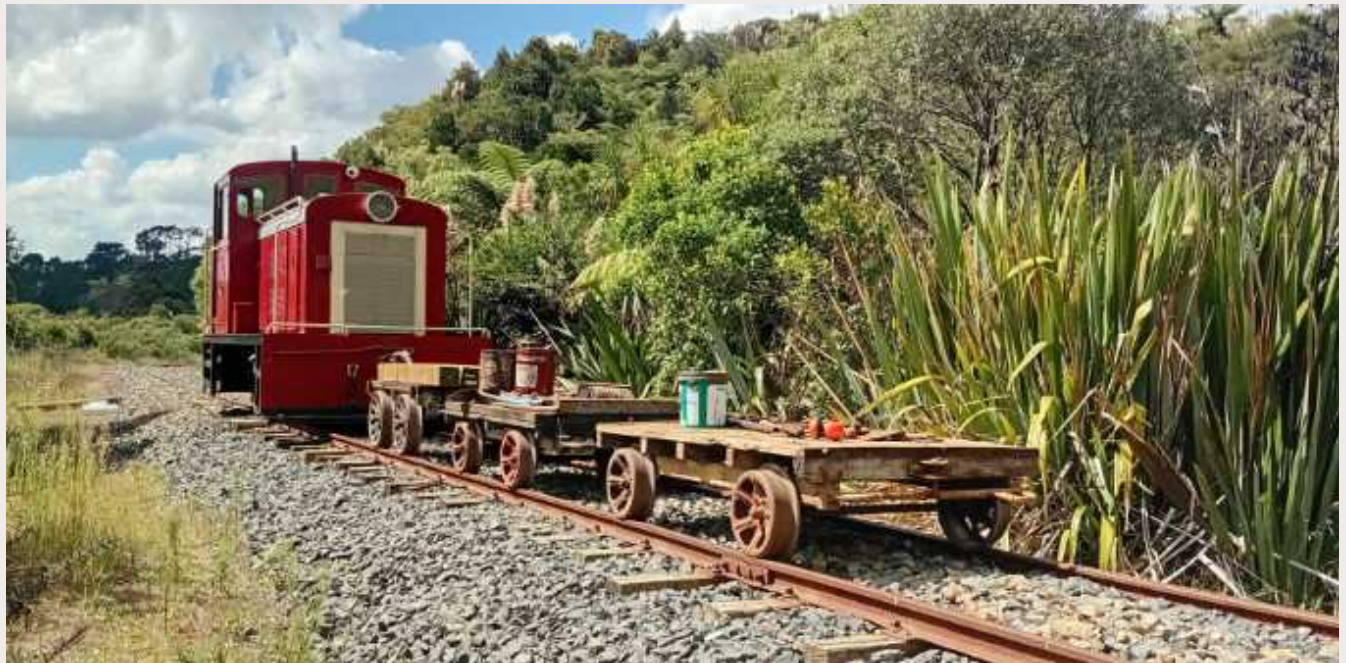
Above: Track work up the line near 1850m (Richard E)
