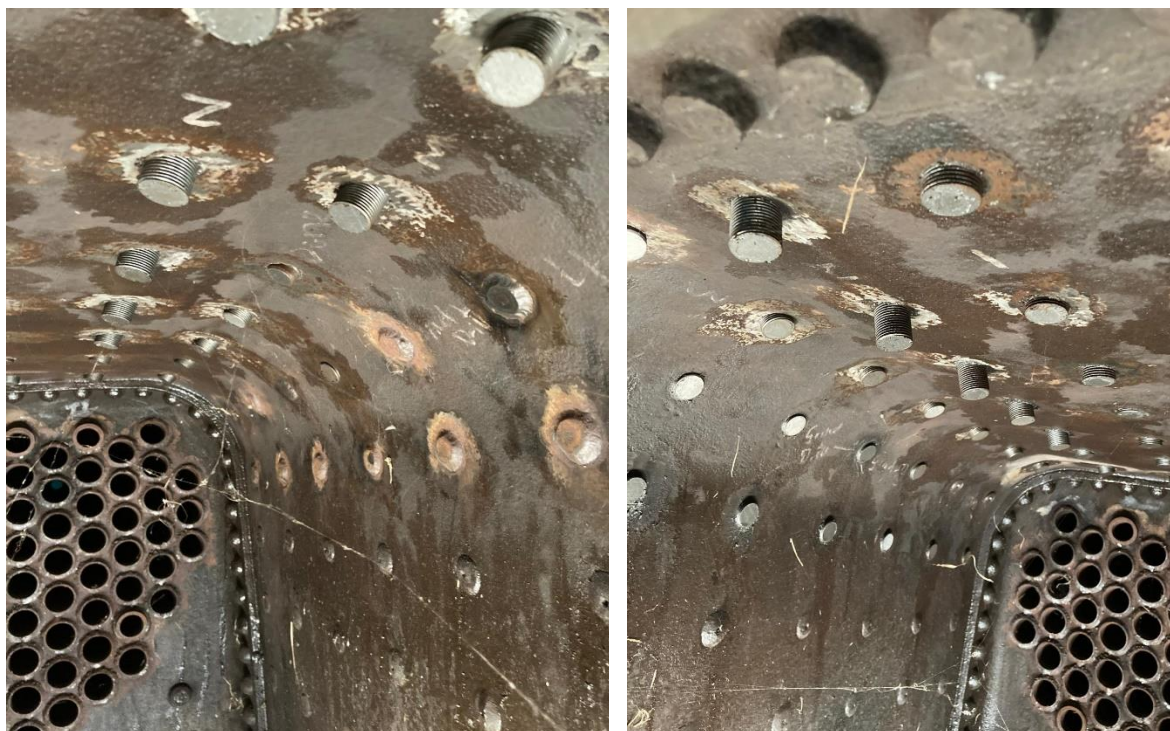
The Heisler firebox in 2022 – not far from completion and the money was donated 2 years ago to finish the job (C.Mann)
