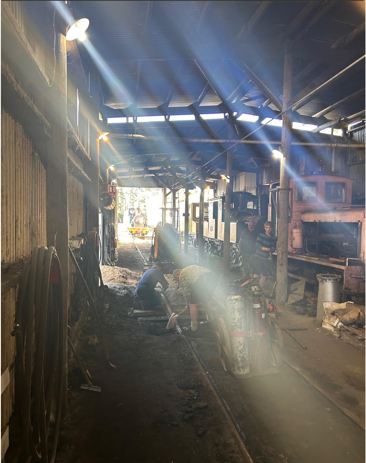
Loco shed view - track work underway (Chris M)
