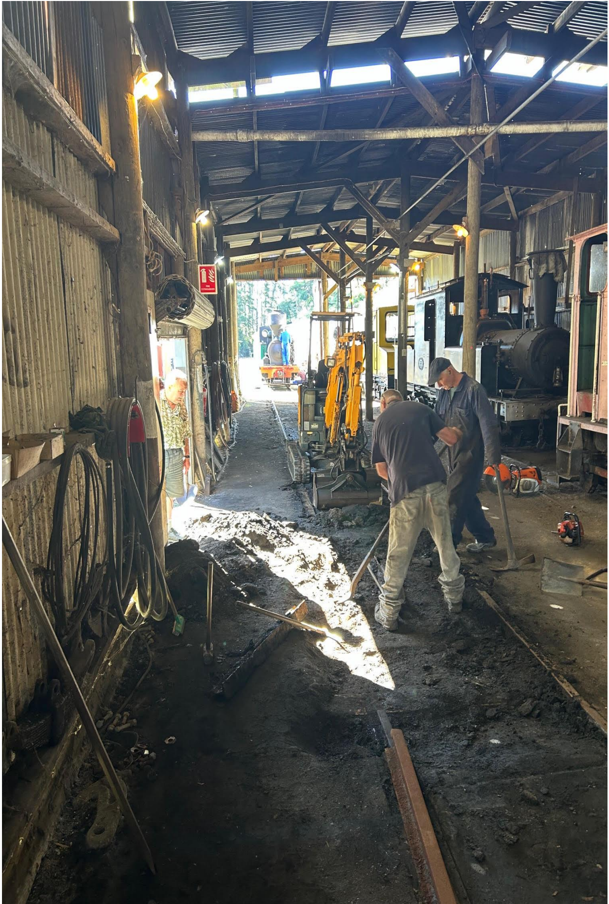
Trackwork in the loco shed (C.Mann)
