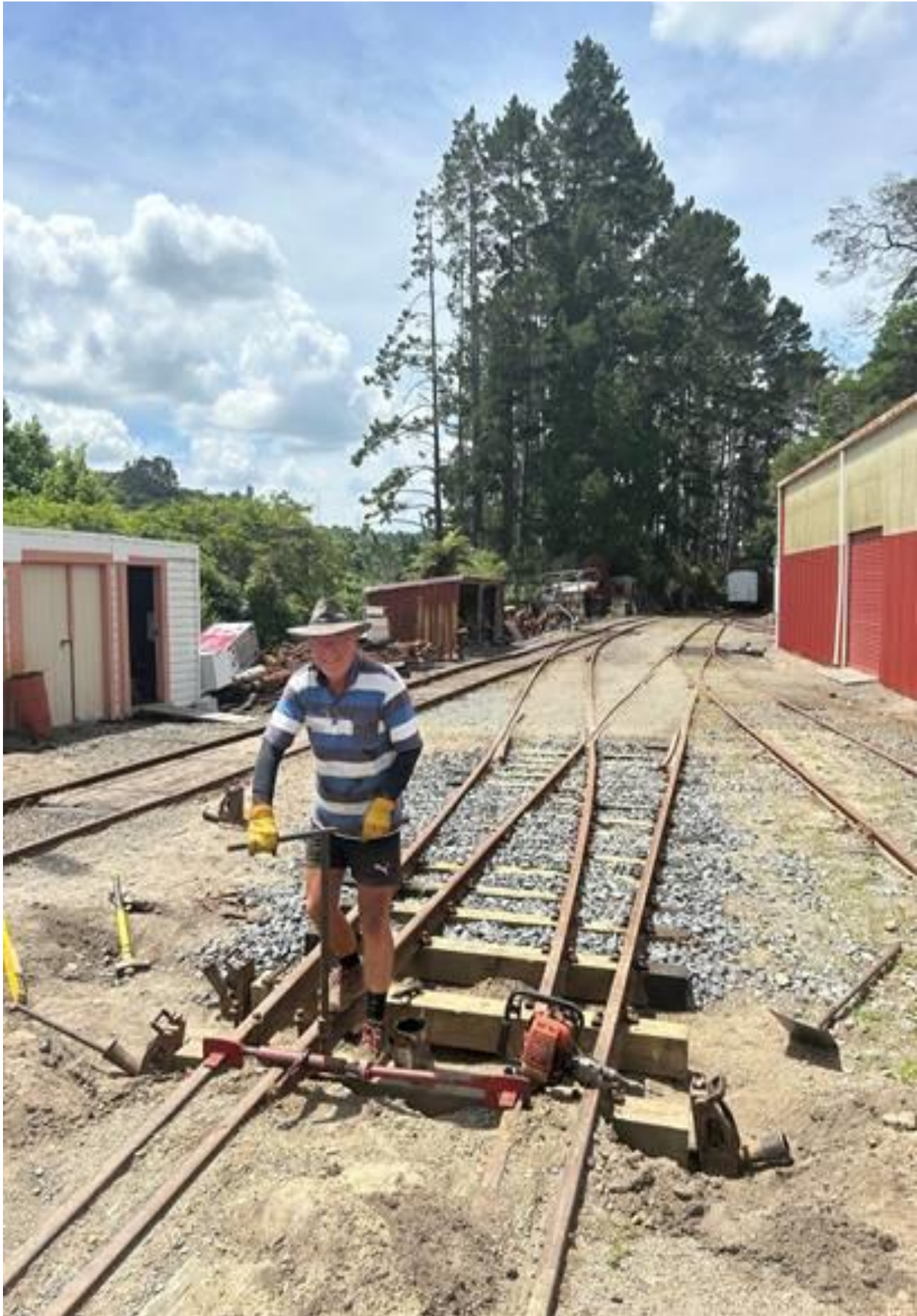
John S repairs a point in the PJ yard
