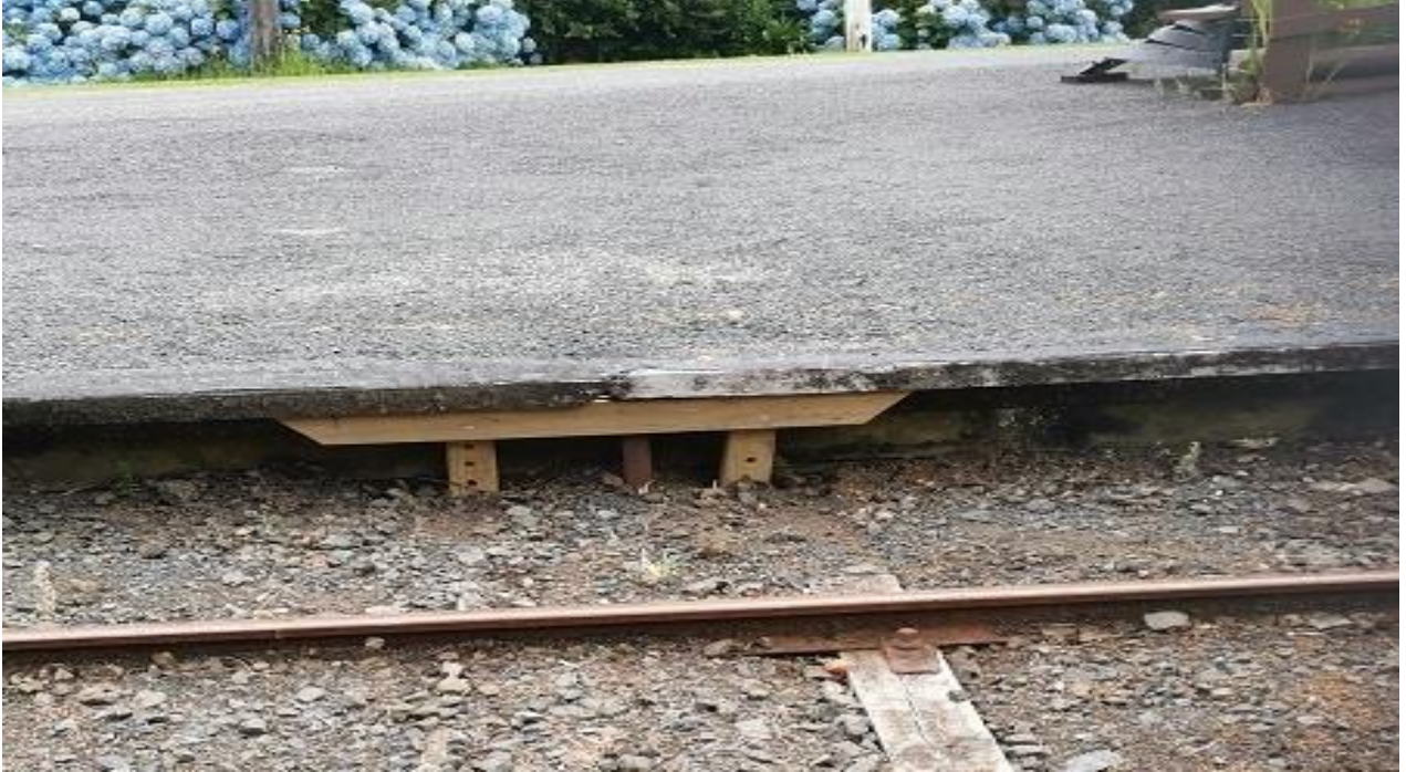
Bruce McL has been repairing the platform edge (Trevor W)
