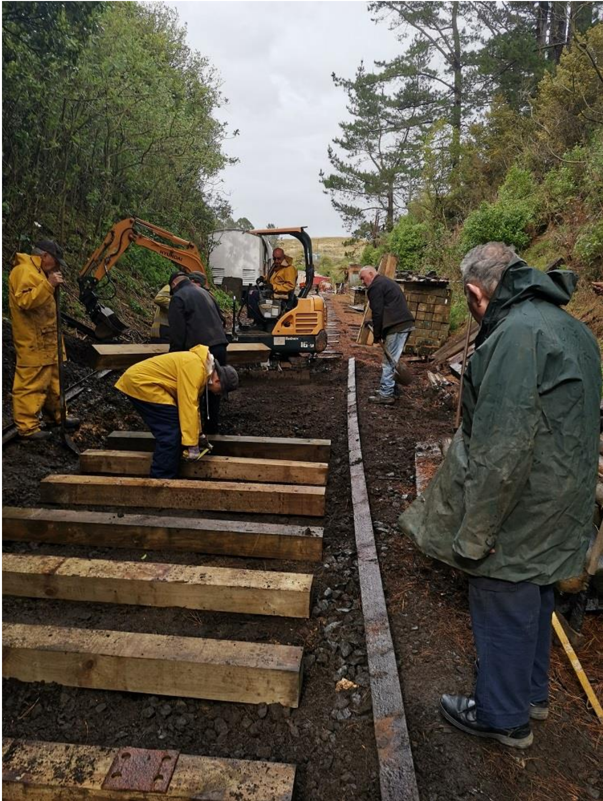
New sleepers being laid (T.Willmot)
