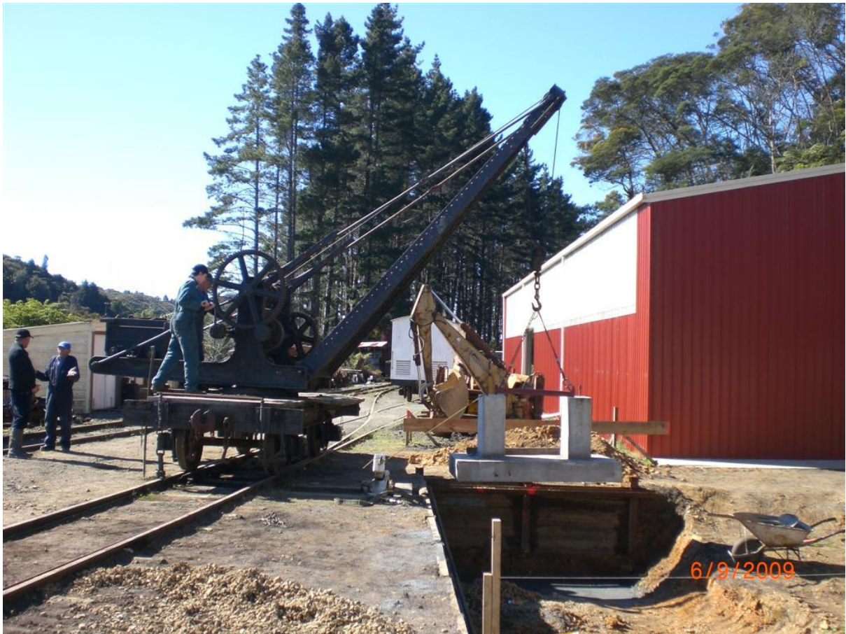
The pit under construction many years ago (C.Lucas/R.Stratford)
