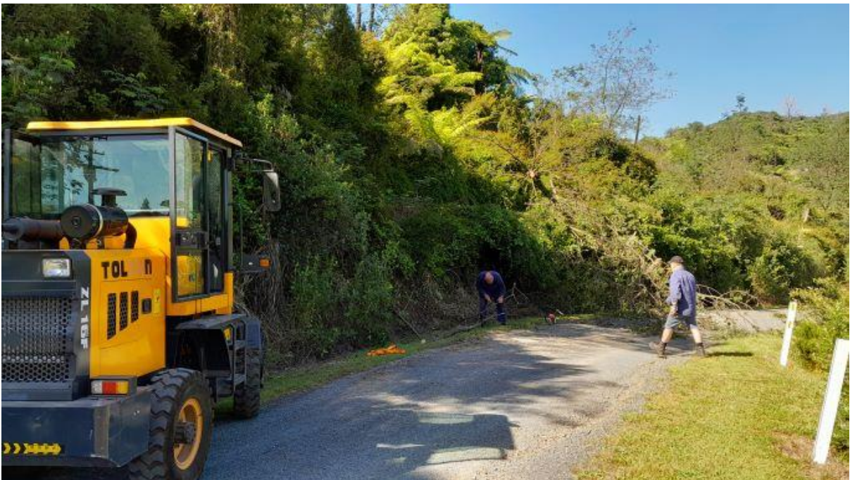
Clearing up the driveway (Photo: J.Soffe)
