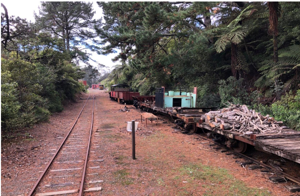
View of the top of the PJ yard (C. Mann)
