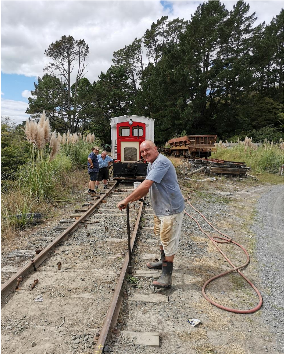
Early work lifting the old track (T. Willmot)
