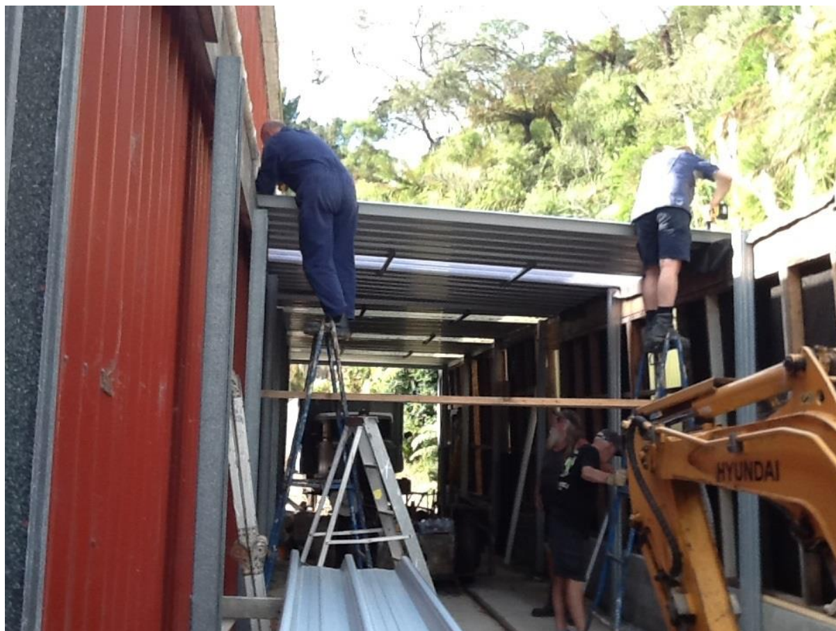
Work on the roof of the lean-to (I. Jenner)
