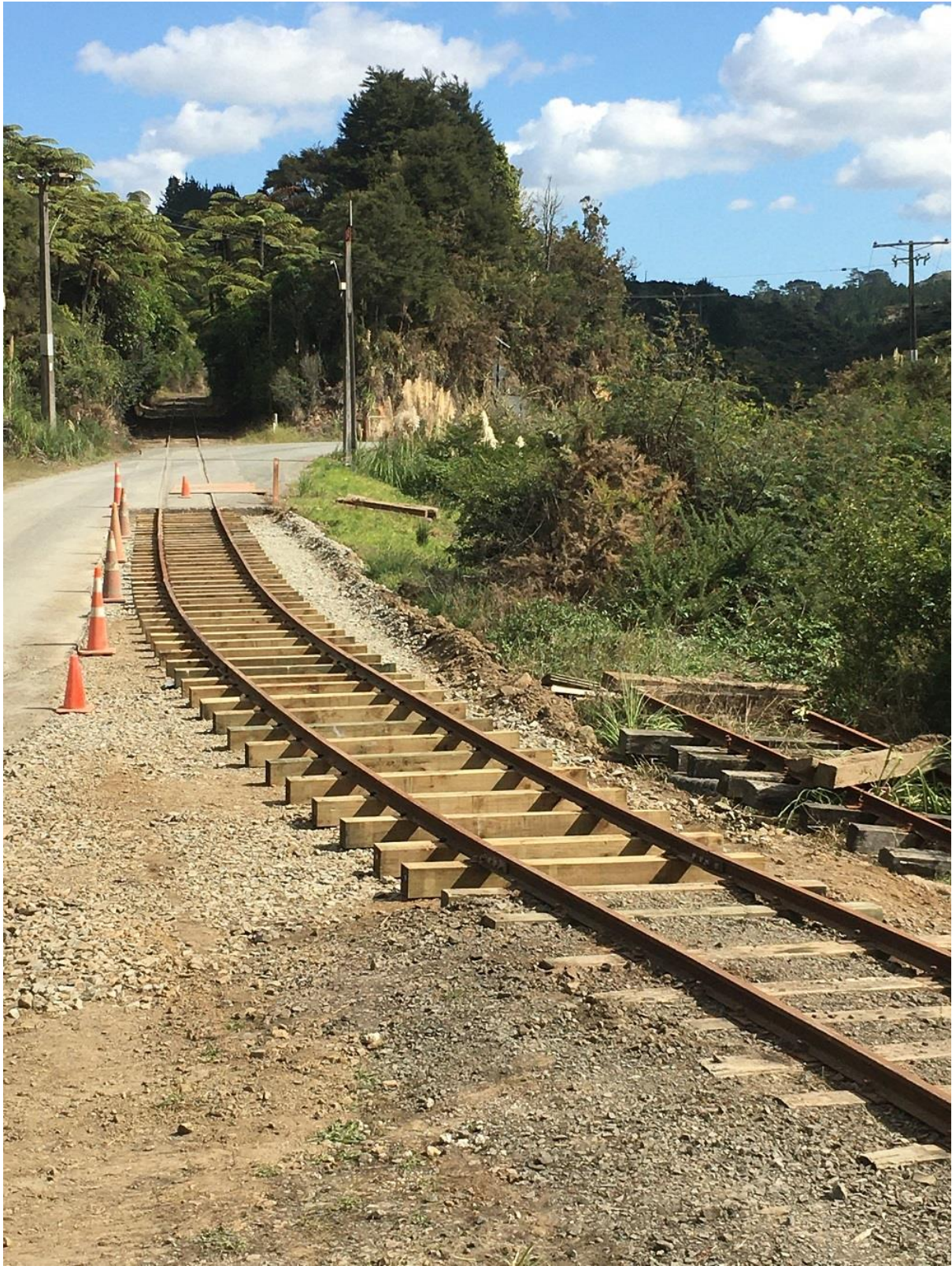
The new track at the crossing (P. Cairncross)
