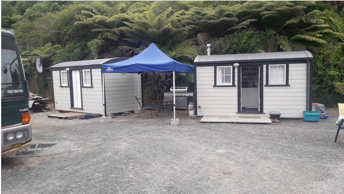
The two new recently built huts now on site (T.Townsend)
