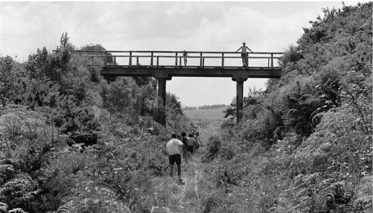
Hangapipi road bridge 1979 (J.A.Terry)
