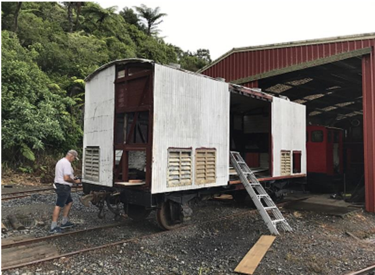
Bruce working on the Xp wagon outside the woodwork shop (E. Baptist)
