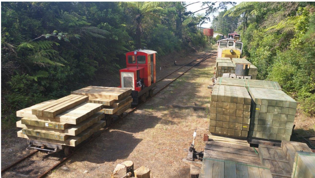
The Planet propels a load of sleepers up the main line whilst more stored sleepers and Tr436 are seen on the siding (J. Soffe)
