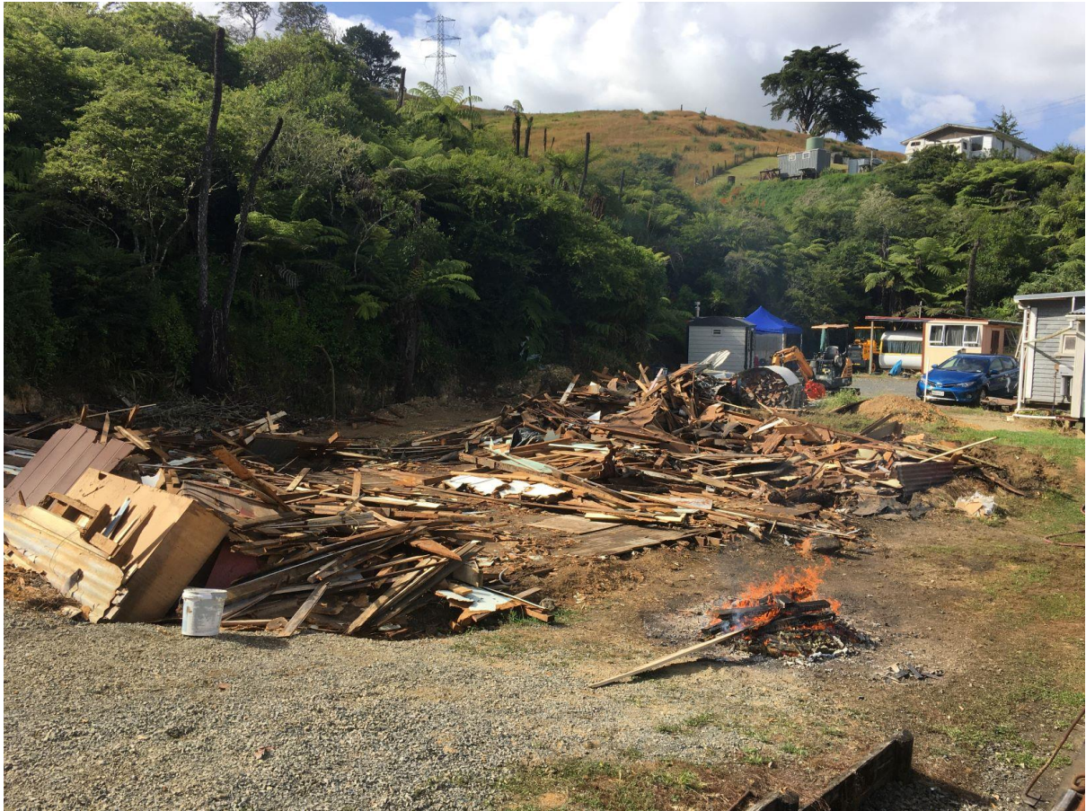
The old hall further demolished (P. Cairncross)
