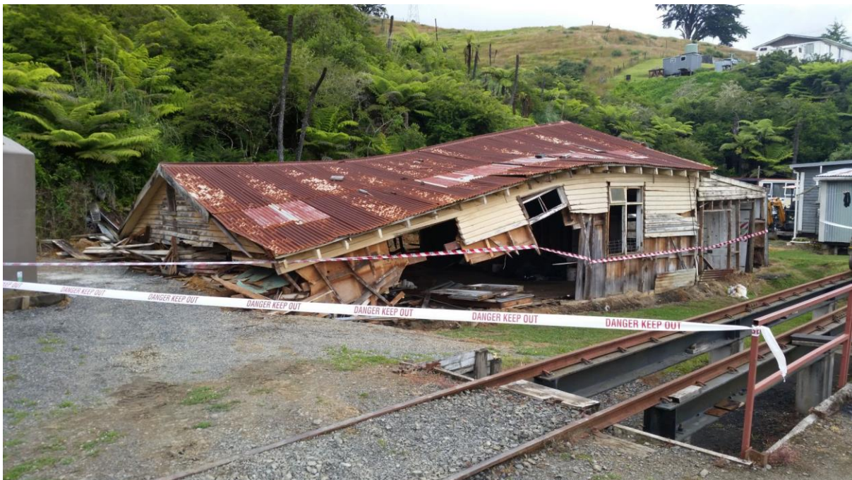
The old hall partially demolished (R. Beaumont)
