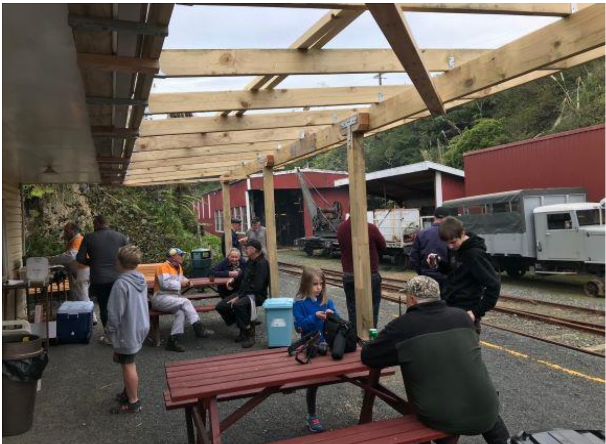
The new awning takes shape. (Photo: E. Baptist)
