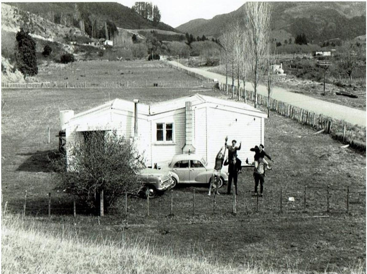
Members of the BTC camped in a shearing shed at Ongarue in the 1960's. The mill was in the centre distance and the Price "E" is visible off to the right (image: I. Jenner)
