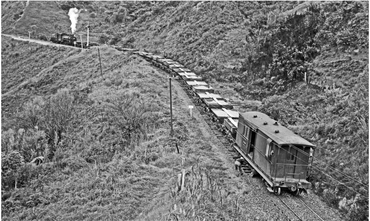
In 1949 this train was ballasting our line....a ballast plough in the foreground (photo Len Hostick from the John Agnew collection)
