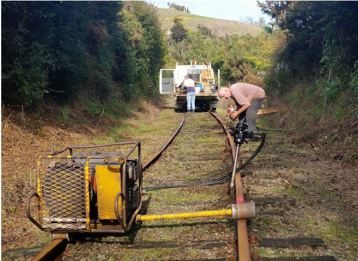
David Mann hard at work using Dean's equipment to refurbish the track (Image: J. Soffe)
