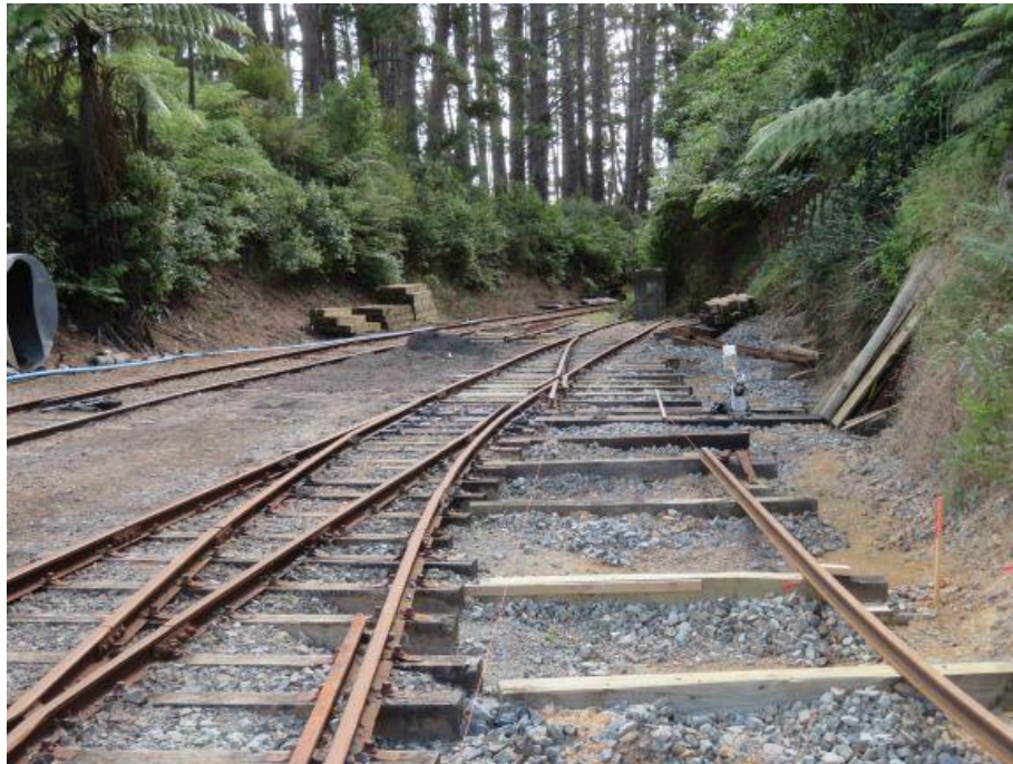
Following a couple of successful working bees organised by Trevor Townsend, the new siding for the battery electric loco approaches the point on the right hand side of the picture (R. Ellis)
