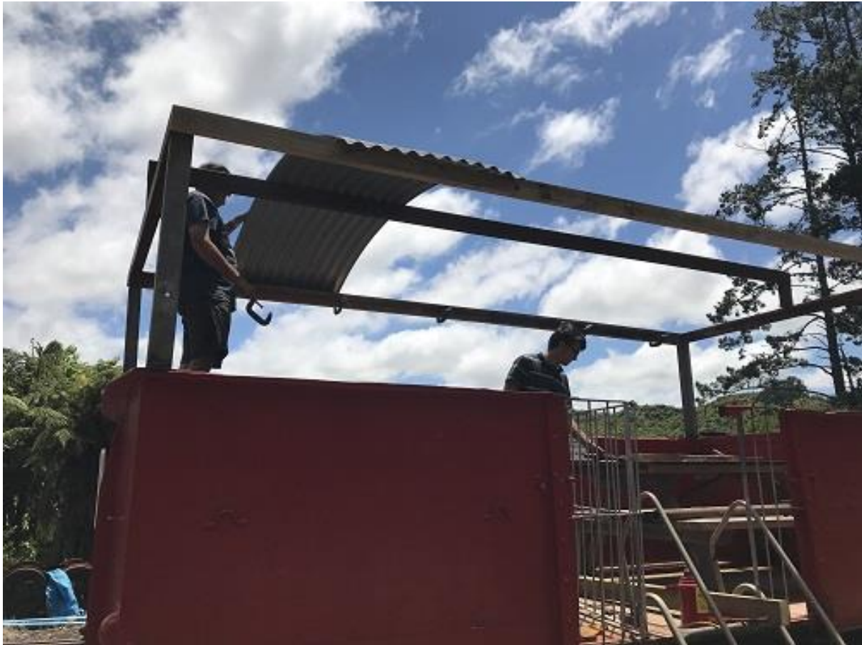
Work on the LA17313 wagon roof proceeds (E. Baptist)
