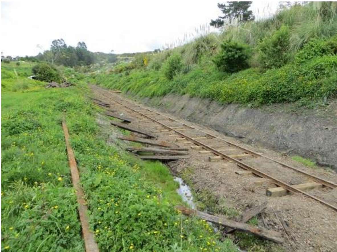
Sleepers replaced by Dean, assisted by Dave Mann at Glen Afton (B. McLuckie)
