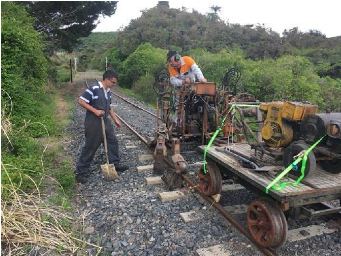
Jordan & Pete tamping near Hangapihi Road (P. Cairncross)
