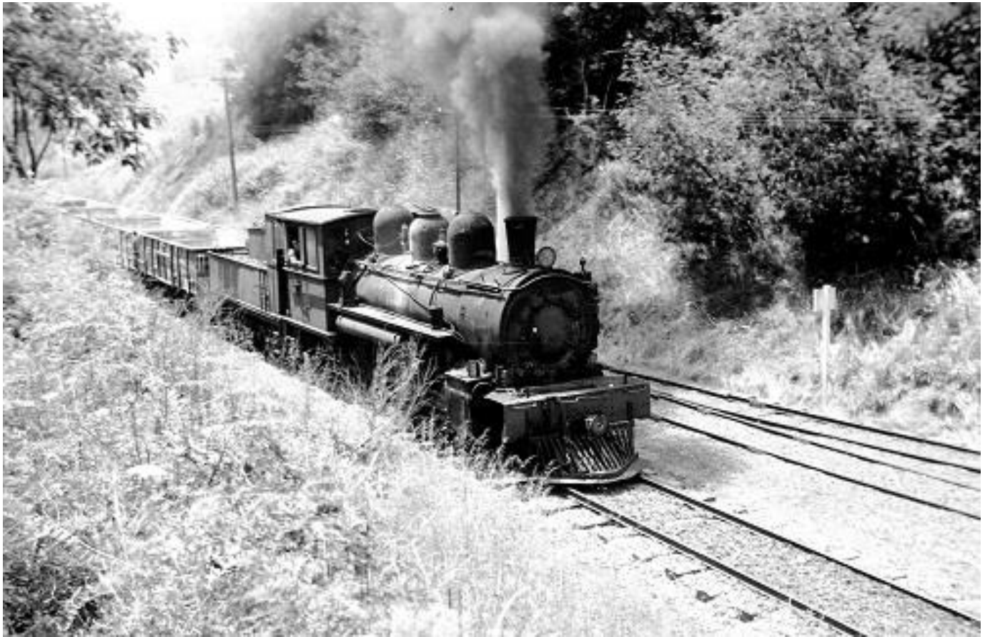
Blast from the past: Bb636 at Pukemiro (image Trev Terry)
