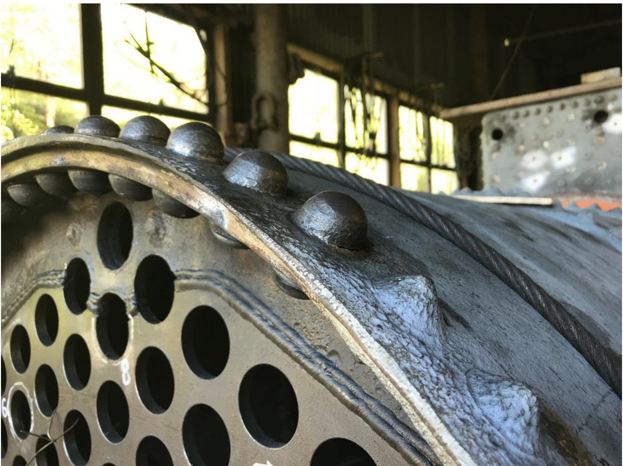
The Climax boiler is being worked on again – this close up shows the previous work done on the tube plate and the wasted rivets.
