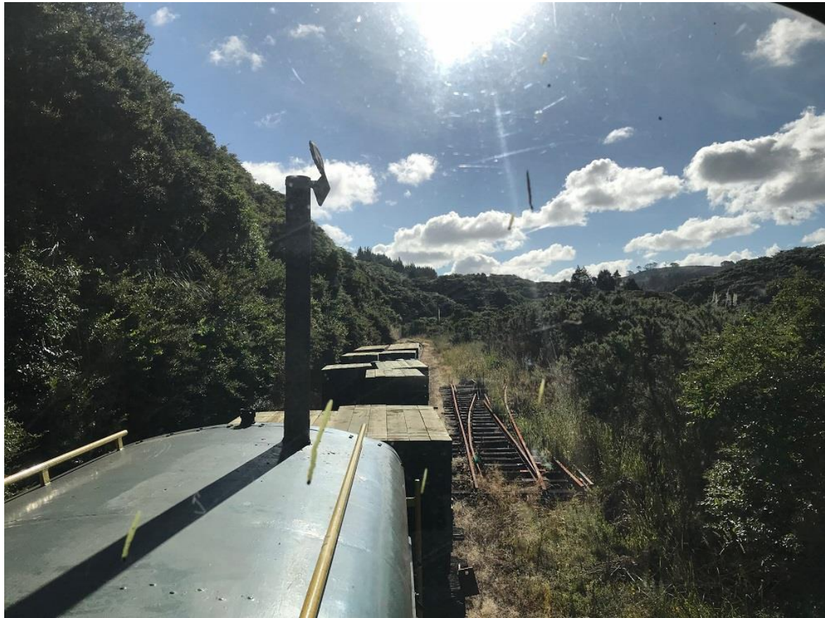
Delivering the sleepers to a “safe place” up the line....
