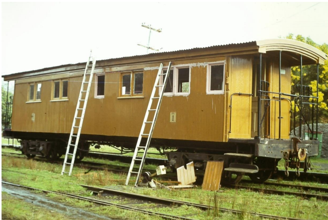
In 1985 Richard Ellis & Carol Mann spent a week finding and installing the “missing windows” in the Mines car.
