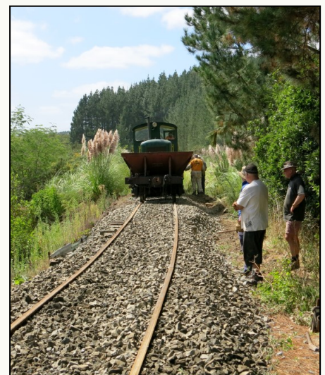
Before/After dropping and spreading ballast. (Image E.B.)
