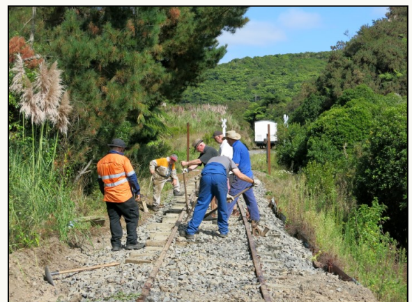
Fixing the Hangapi Road track slump together. (Image E.B.)
