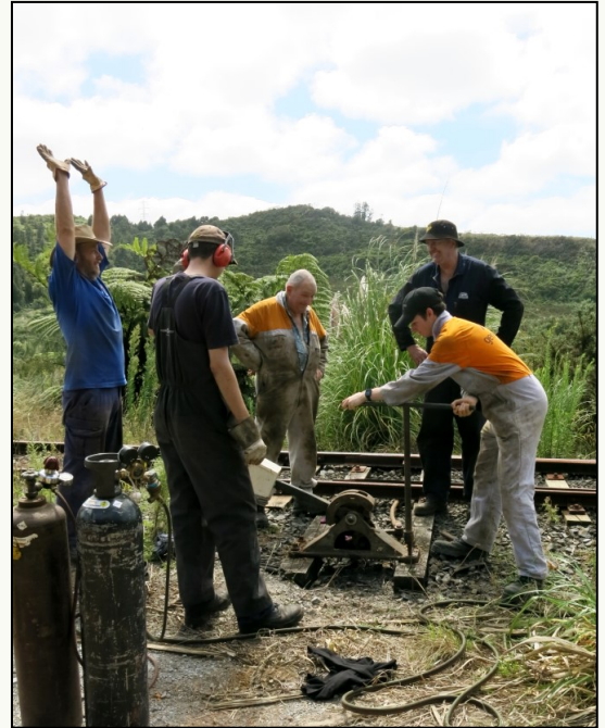
A new, hopefully "theft-proof" points base and lever were also installed while down the line. This image is a particularly rare sight, your editor at work! (Image Guy Coker)
