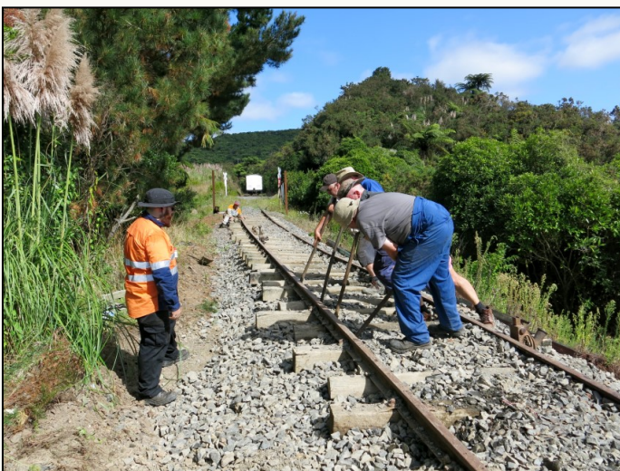
Heave-ho! Fixing the Hangapi Road track slump.(Image: Elliot Baptist)
