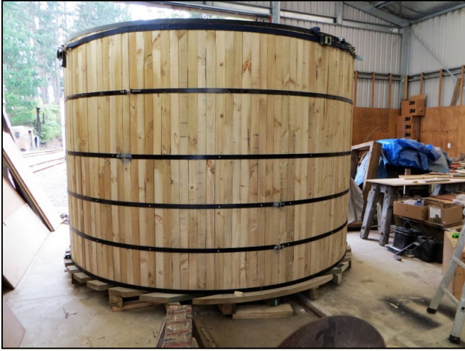
Water tank surround finished and ready for painting (Image: B.M.)
