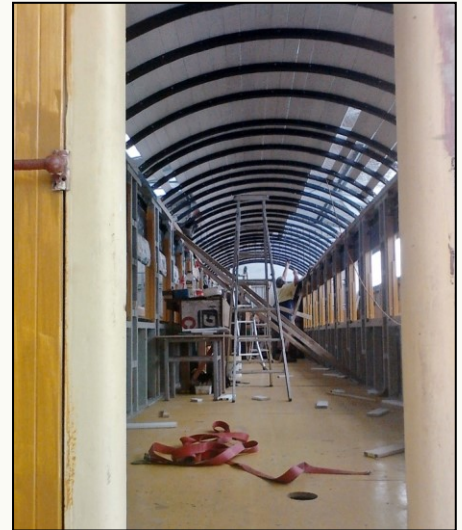
Roof-in-progress. (Image: R.E.)
