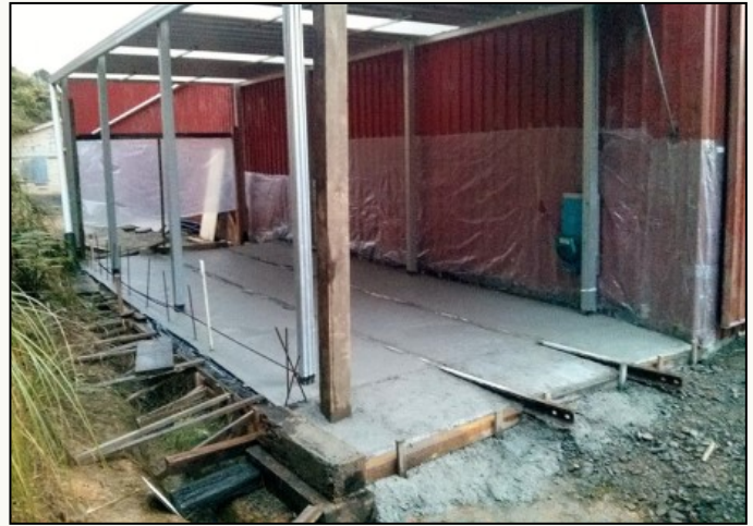
The finished pour, cemented forever more. Photo: Lindsey McLeod
