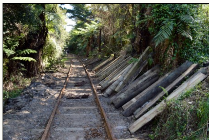
Once cleared the track can be re-sleepered
