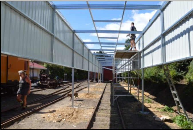
Rapid construction underway by Totalspan
