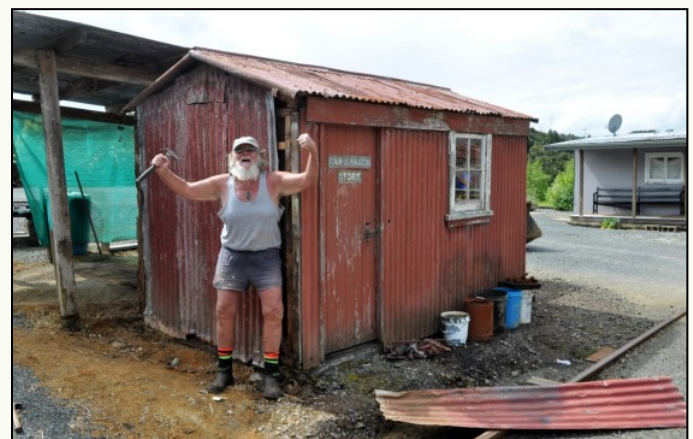
The day the wall fell (thanks to some handy hammer work)
