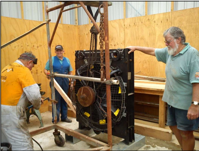
The fan cover on the Ds radiator needed a bit of ‘persuading’ to fit back on. Here CJ (on left) is about to gas cut a bit off so that the bolt holes will line up. Also in the picture is our new member, Russell (on right), and Bruce (in the back).
